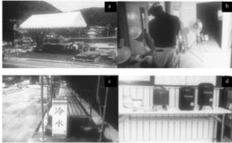
Fig. 1. Some measures taken at the subjective construction site.
